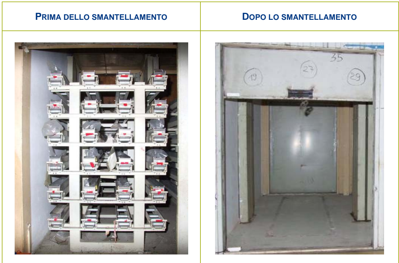
Figura 2-6 - Smantellamento racks (locale A121)
