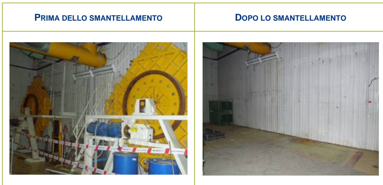
Figura 2-15 – Smantellamento blenders (locale A107)
