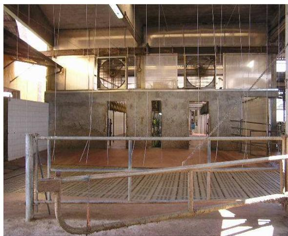
**Fig. 2 – Ventilatori in sala mungitura**
