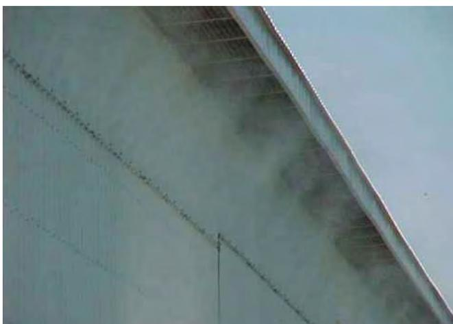
Foto 12: raffrescamento mediante fogging cooler
