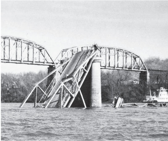
Silver Bridge Ohio, 1967 stress corrosion and corrosion fatigue
