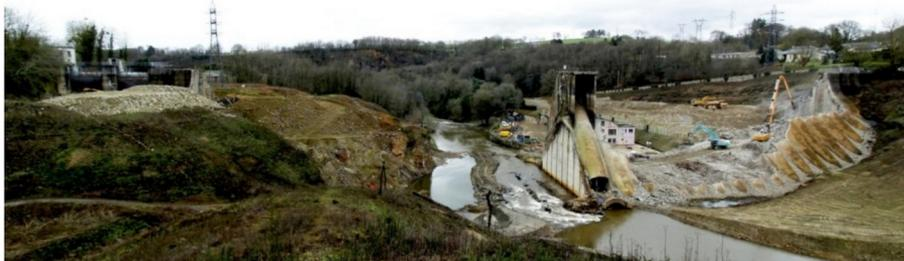
Vezius dam 13 January 2020 : 80 % of the 36 m high dam removed © DDTM50 in coop. with ERN
