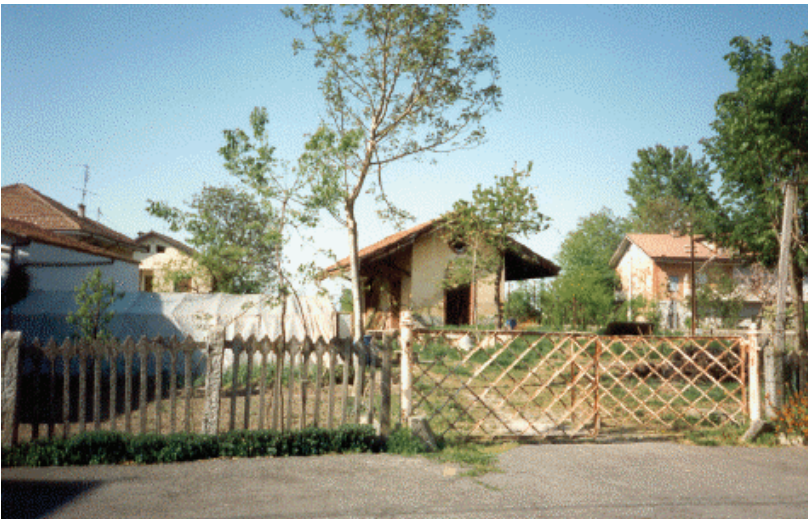
FIGURE 76-77: Magazzino Merci al Km 16+221
