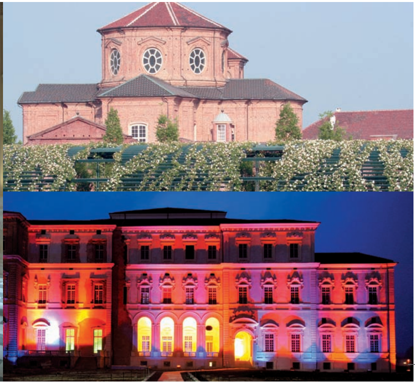
Left: Main gallery Top: Pergola S.Ubaldo Bottom: Royal Palace Source: "Progetto La Venaria Reale"
