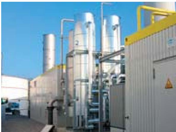
Figura 27 - Impianto PSA a Mühlacker [CarboTech (2008)]
